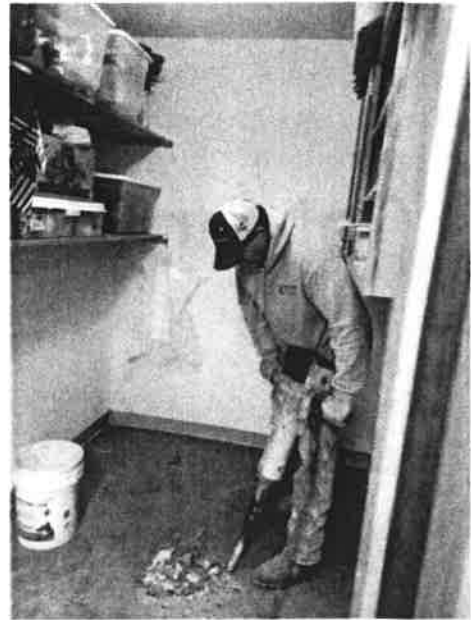
Matt installing the sump pump
